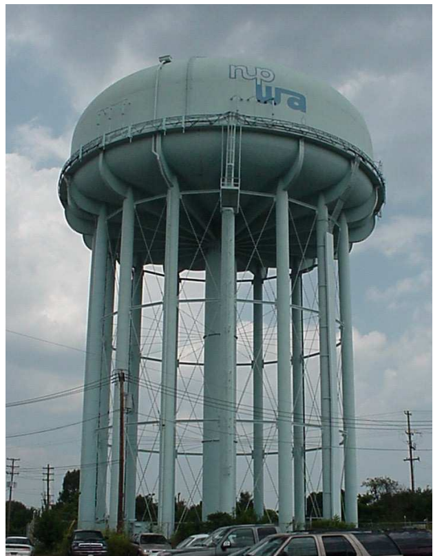
Elevated tank in the North Penn system
