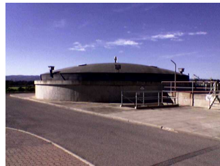
Organic Sludge Digester
