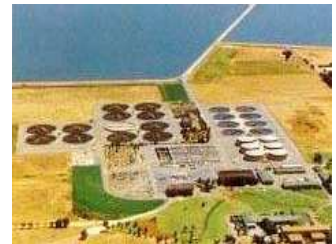
Bolivar Wastewater Treatment Plant
