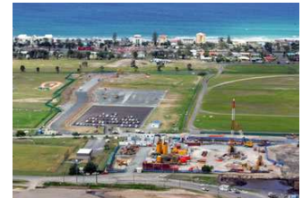
Tugun - Planned site for desalination plant
